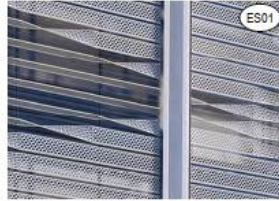
EXTERNAL SCREENS PERFORATED CUSTOM LOUVRES
